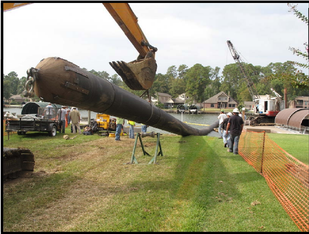
Horizontal Directional Drilling Shore Approach
